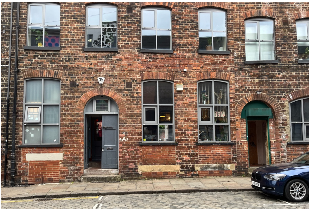
Figure 12. Wharf Chambers exterior, Leeds (June 2023)
