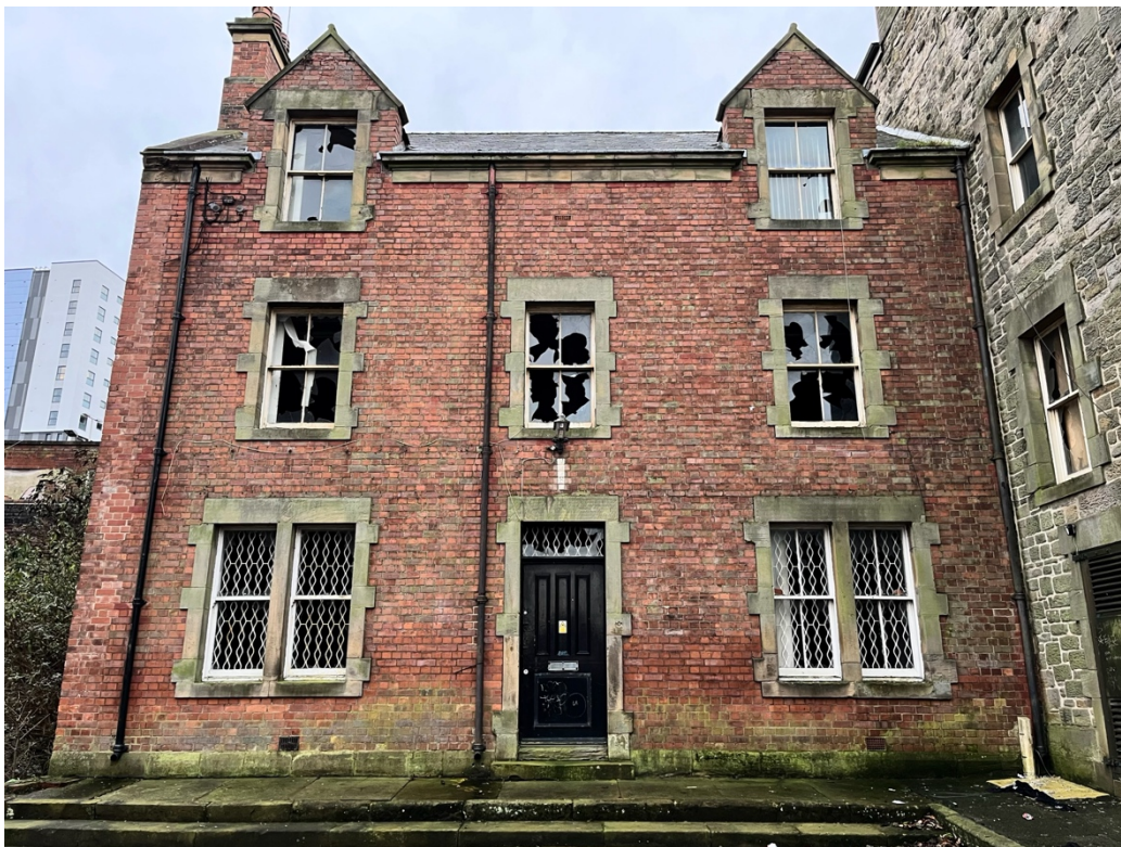
Figure 40. The former Old Police House (December 2025)
